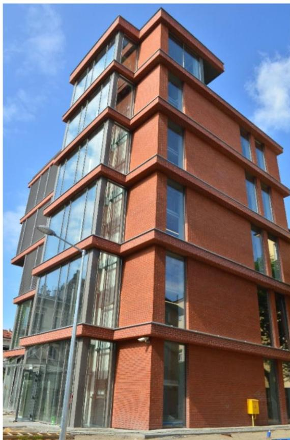
The innovative building is situated on the University campus in Warszawska street. It has 5 floors (built area is 258,41m<sup>2</sup>, utility space is 1039 m<sup>2</sup>, the front elevation is 17,02 m wide and 19,24 m high). It is a slab and column construction with self-supporting external walls and glass elevations.
